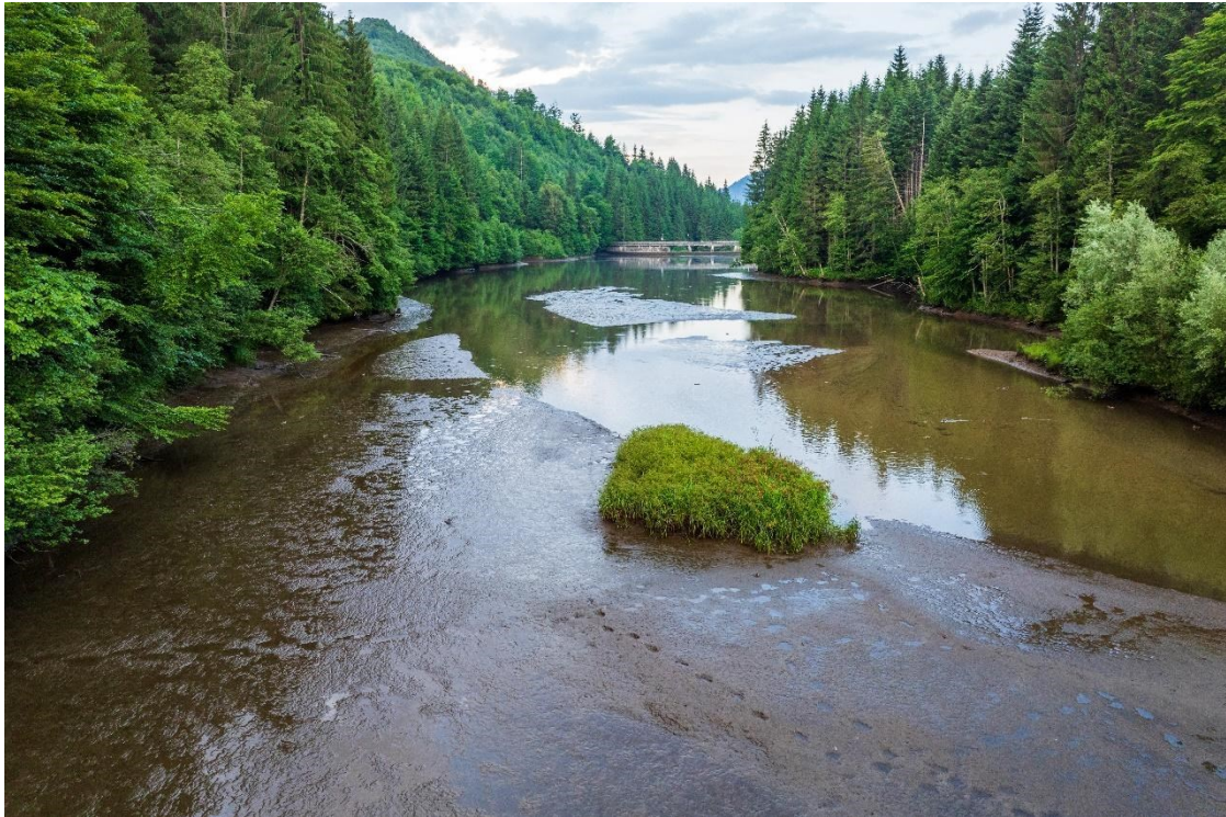
Figure 2. Trapped sediment upstream a dam at Valsan River © Dick Harrewijn
