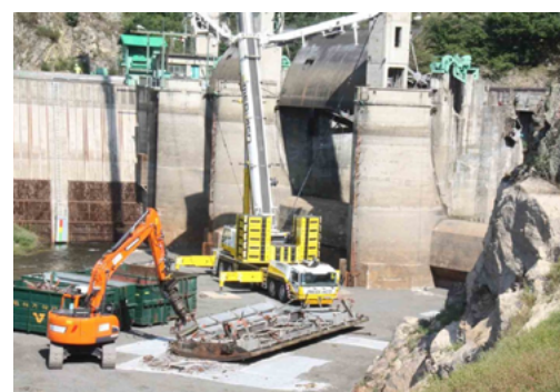
← Removal and destruction of valves on the Poutès
