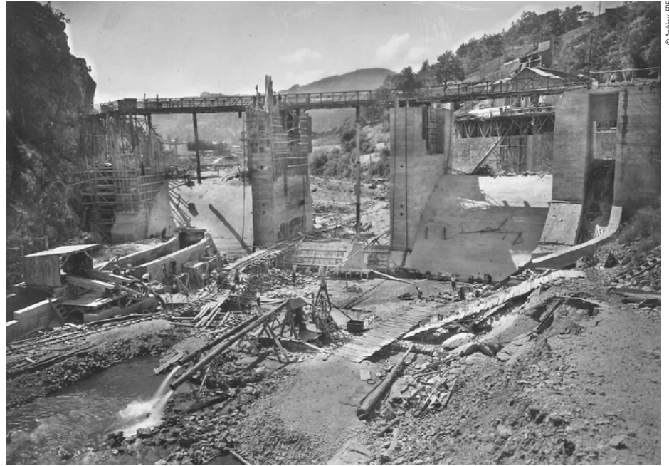
↑ Construction of the Poutès dam
