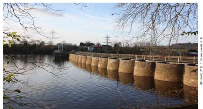
↑ Reservoir lake of Vezins dam
